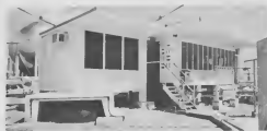
Gasoline Pumphouse Office with addition at left. Oficina di Gasoline Pumphouse cu adición na robes.
